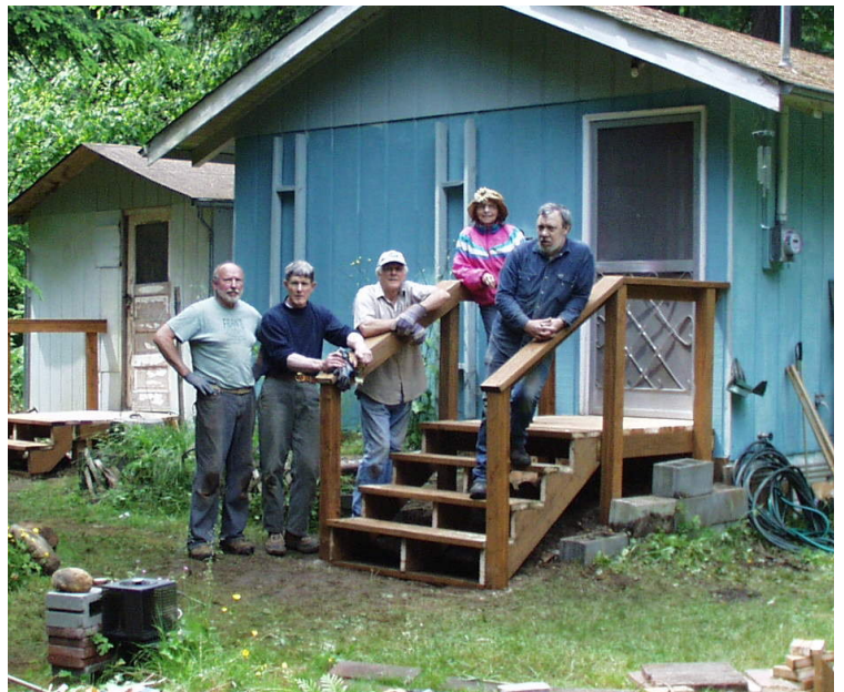
After with porch, steps and railings.
