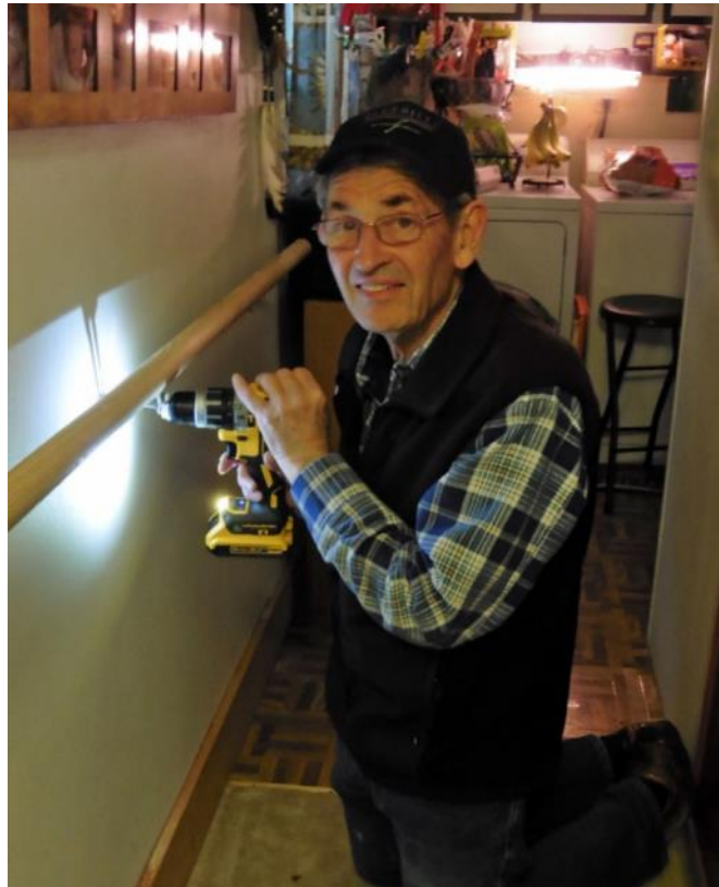
David Grellier Securing Hallway Railing
