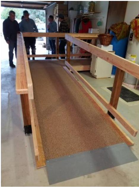
This ramp is built inside the garage.
