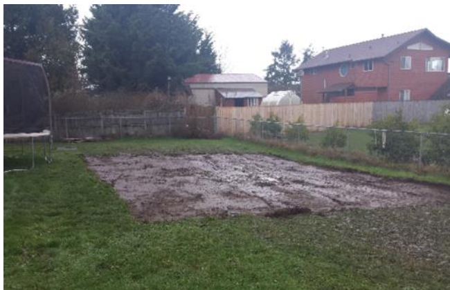
The 32 foot by 24 foot area where the Gorilla play set will be assembled
