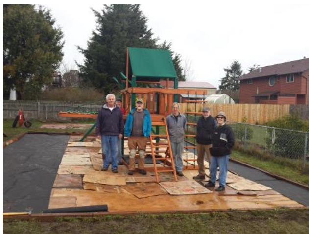
Day Two: Assembly Complete Awaiting delivery of the cedar chips
