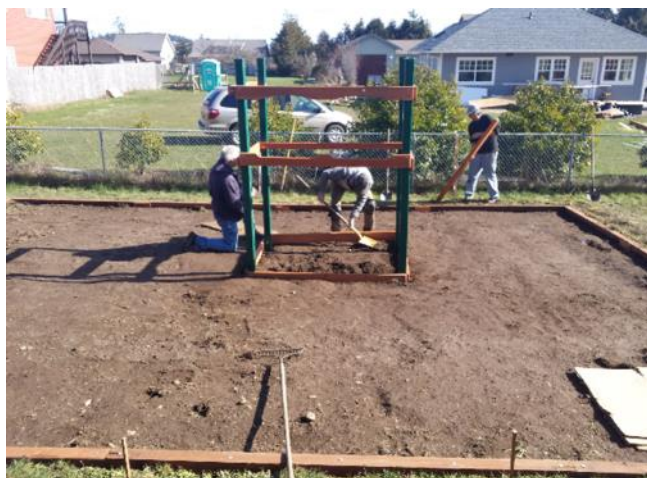
Day One: Assembly Begins Setting and leveling the base.
