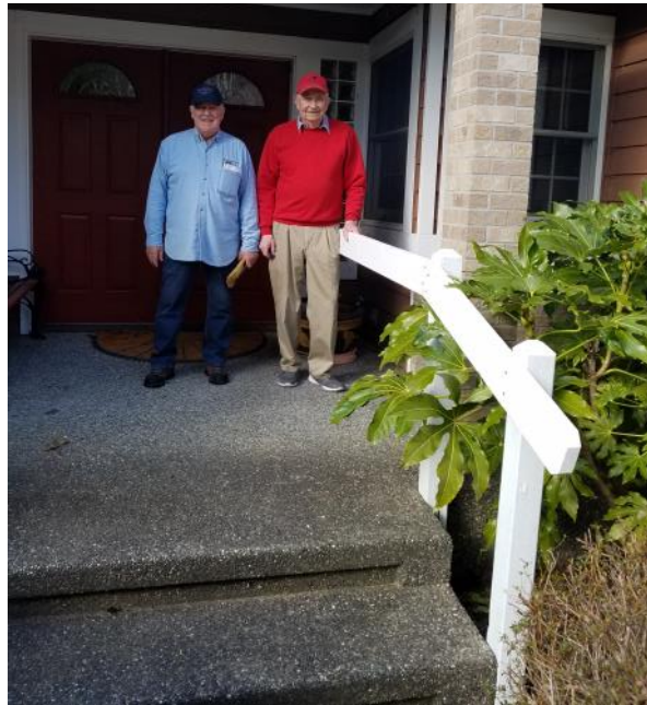
The client for this job had suffered injuries twice, falling from these stairs. David Parish and Myron Vogt shown, photo by Jim Mueller
