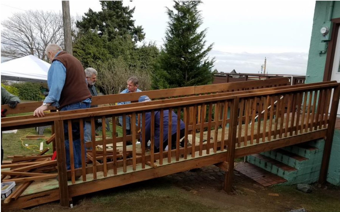
This is a ramp build and thank you card from the recipient. Built on a rainy day in Port Angeles by this crew.
