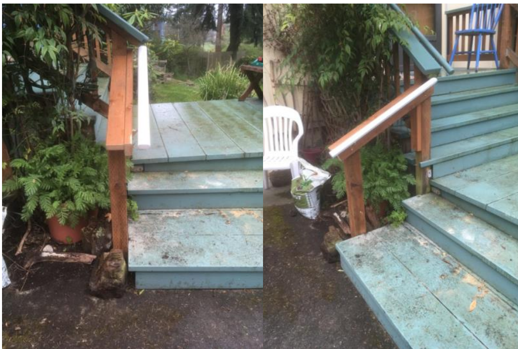
Dan Nieuwsma installed this handrail for a client in Port Townsend.
