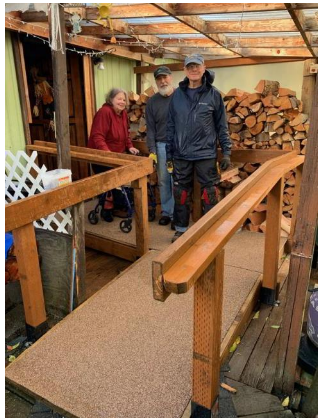
New ramp with platform and handrails. Client on left with Glen Bell and John Fillers
